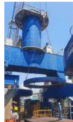
Crane Slewing Bearing renewal
